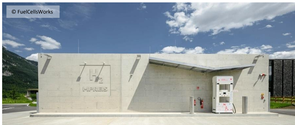
Figure 4 HRS at MPREIS site in Völs, Austria, with a dispenser operating at 350 bar 23
